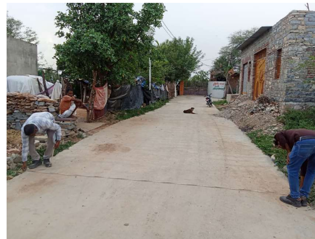
■ Construction of CC Road, Nimbahera
