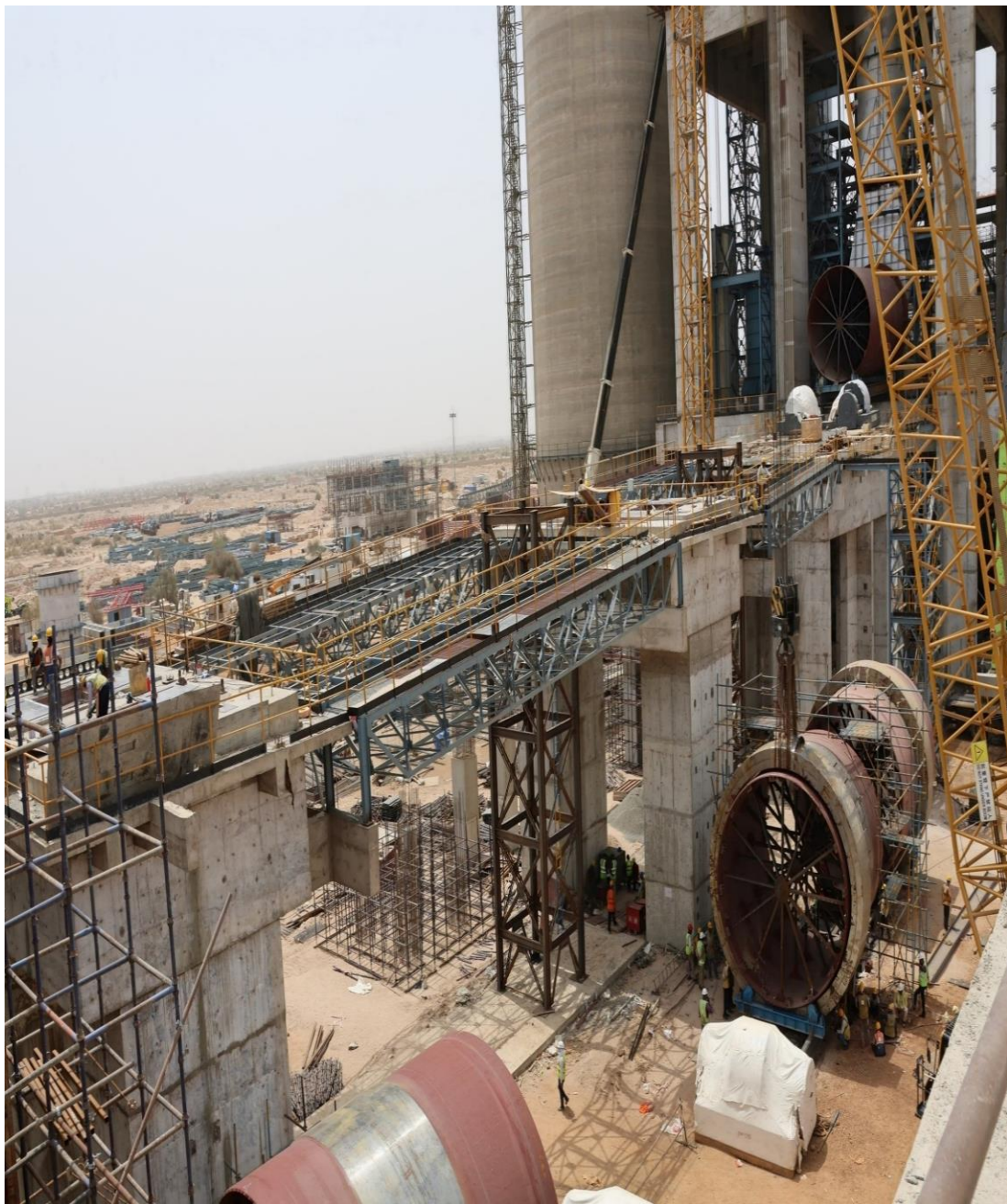
Kiln Line Work
