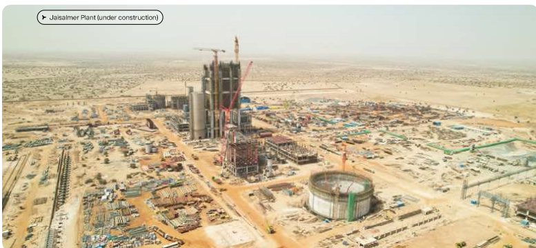
Jaisalmer Plant (under construction)
