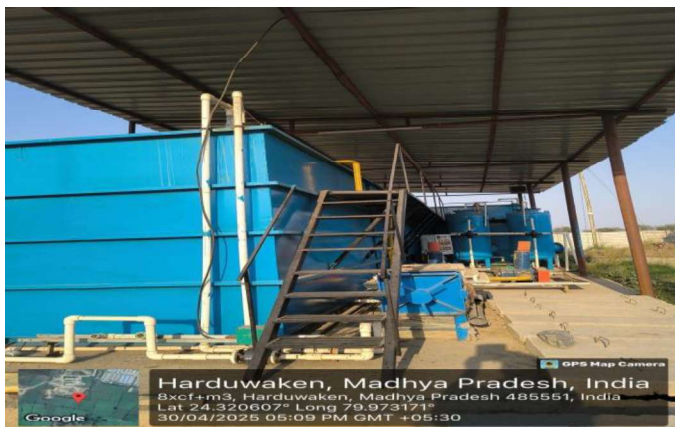
STP photograph 120 KLD & 25 KLD
