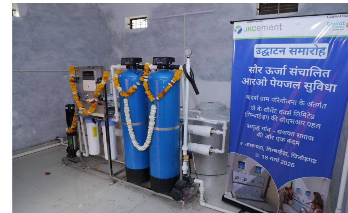
Solar RO Installation at Nimbaheera
