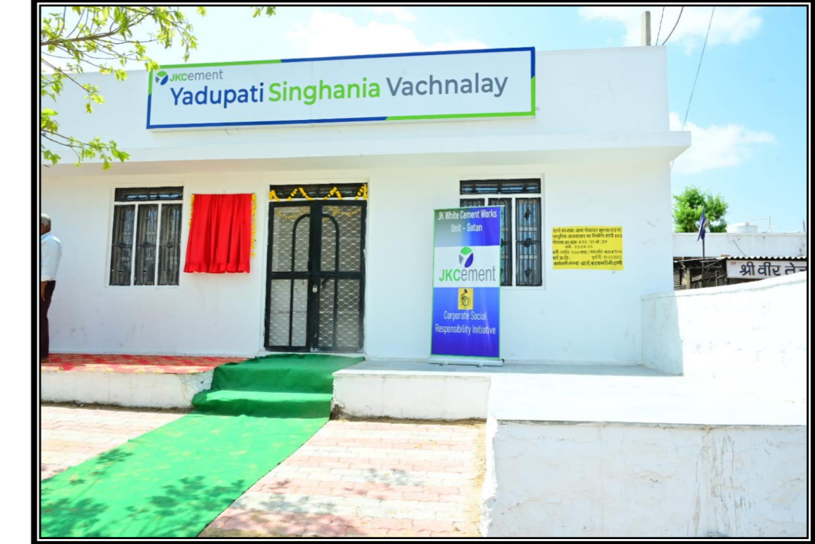
Construction of Vachnalay at Gotan
