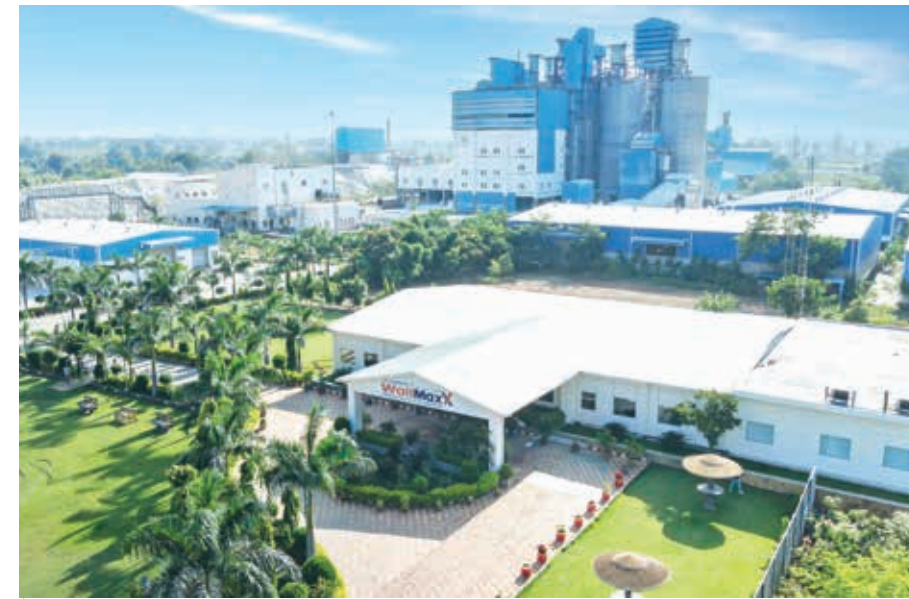
Putty Plant, Katni
