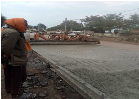
Construction of Village Road at Panna
