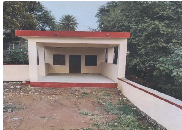
Community Hall Construction at Nimbahera
