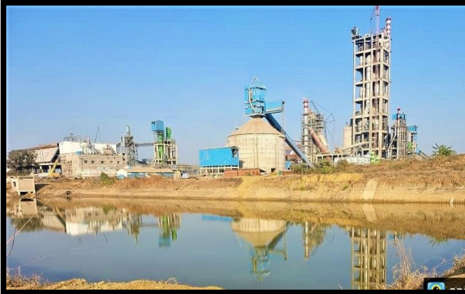
Rain water harvesting pond (30000m3 capacity)
