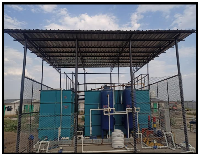
STP With Capacity 300KLD
