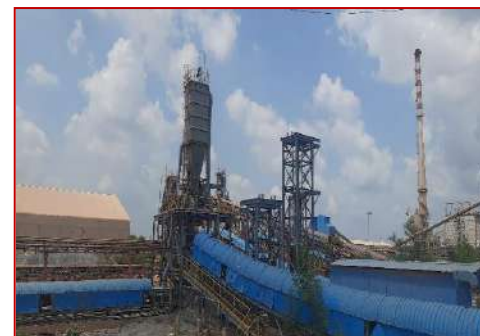
Bag filters installed at material transfer point
