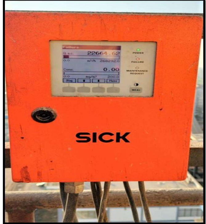
Raw _ Mill Stack Analyser
