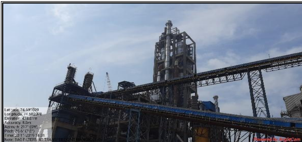
Bag filters installed at material transfer point
