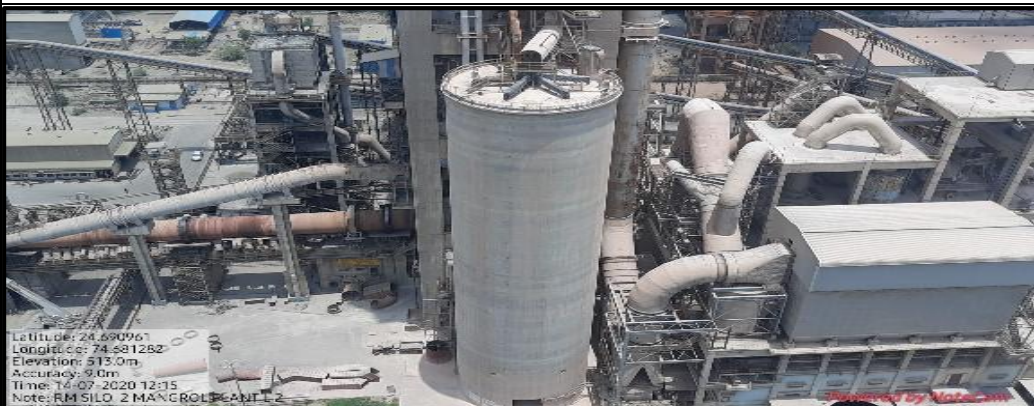
Raw mill storage in CF silo
