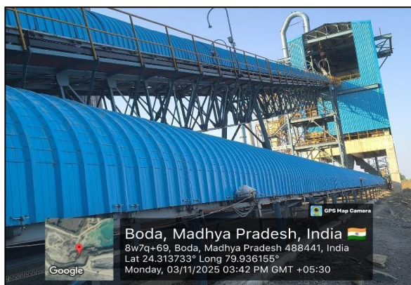
Limestone handling through covered Conveyor belt
