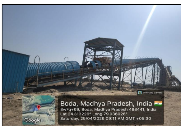
Limestone handling through covered Conveyor belt
