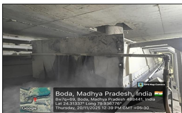
Water fogging system installation
