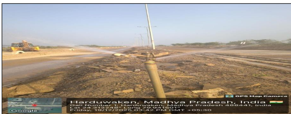
Permanent Water sprinkling at Koni Mine haulage road
