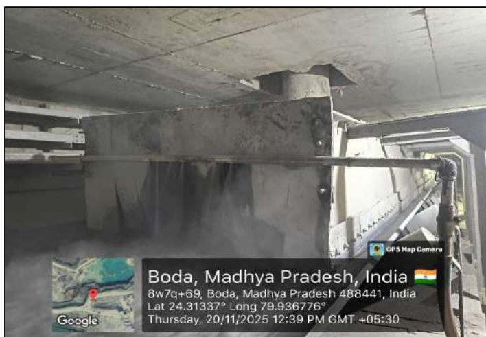
Water fogging system installation
