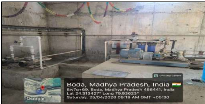
Water fogging system installation
