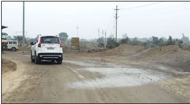
Water sprinkling in Mines haulage road
