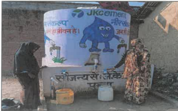
Constructed concrete water tank at Judi Village
