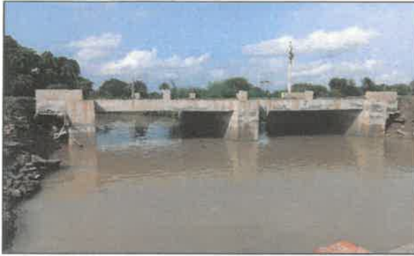
Bridge constructed at Kakra village
