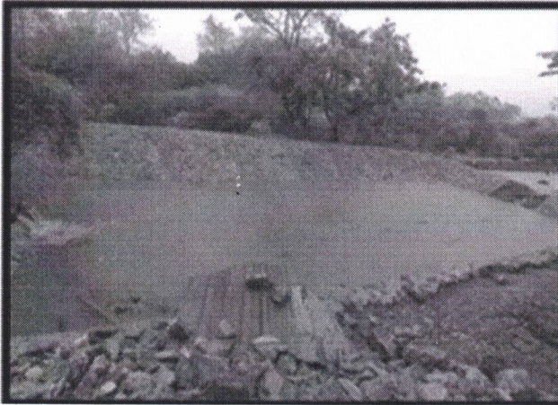
Rainwater Collection Tank at Plant
