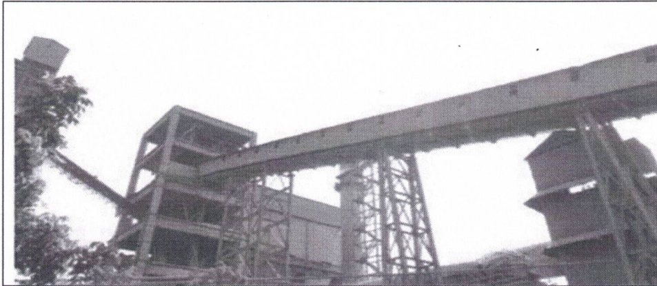
Closed Conveyor System
