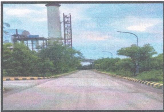
CC Roads constructed in plant to reduce fugitive emission
