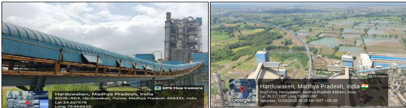
Picture 2- Covered raw material belt conveyor
