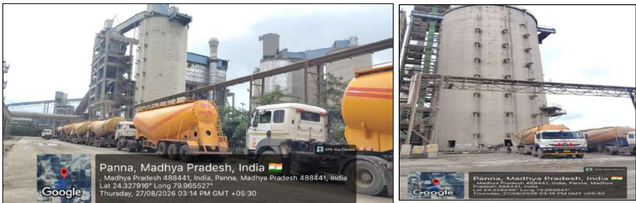
Picture 3- Fly ash & Cement Silos
