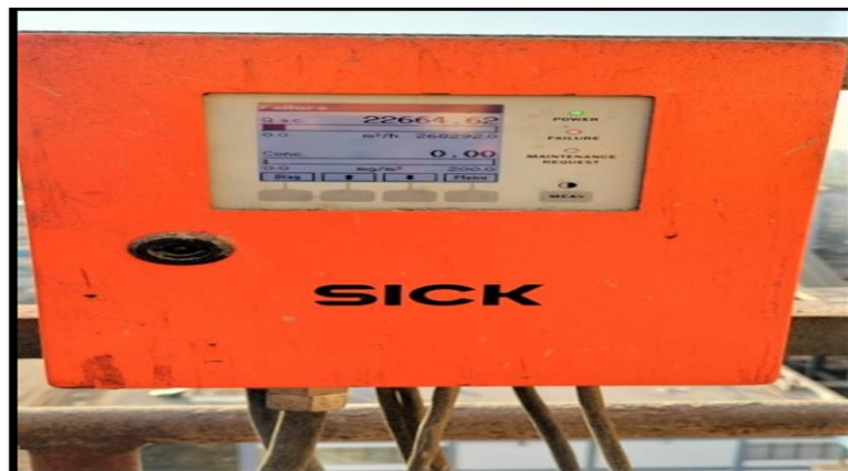
Picture 7- Continuous Emission Monitoring Systems (CEMS) installed and Data uploading in CPCB & MPPCB server
