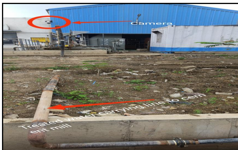
Picture 8- Camera installed at WHRS Treated water discharging point
