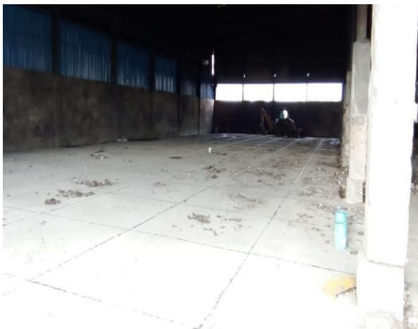
CC flooring in Packing Plant
