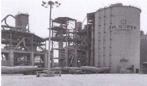
Silo, bag filter and cover belt Pics.
