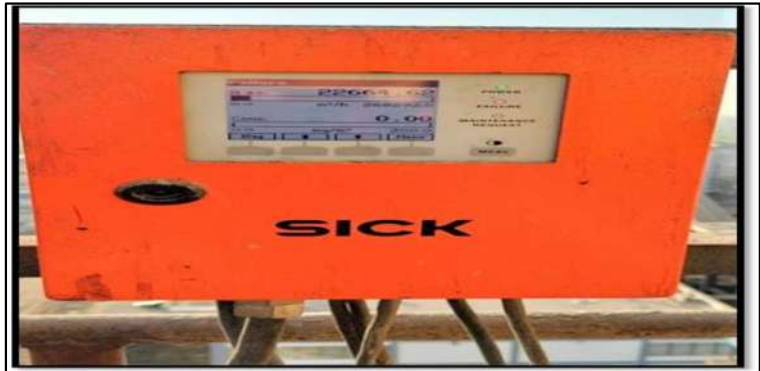
Raw _ Mill Stack Analyser
