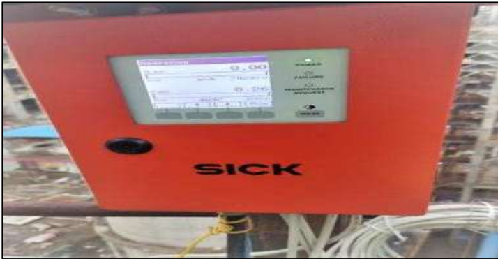
Cooler _ Mill Stack Analyser
