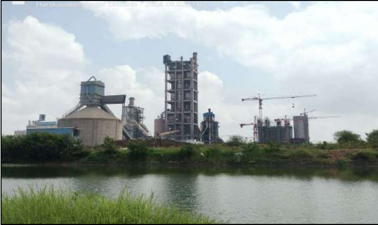
Rain water harvesting pond (30000m3 capacity)
