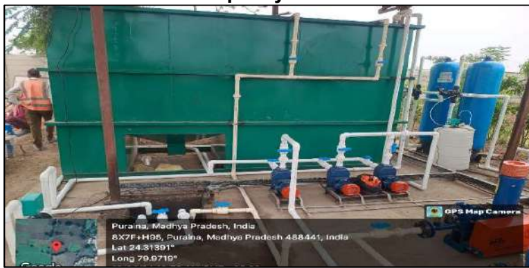
STP With Capacity 25 KLD
