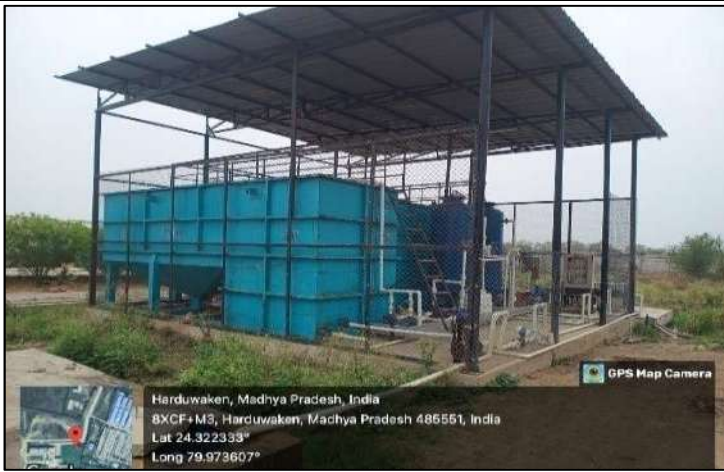
STP With Capacity 25 KLD
