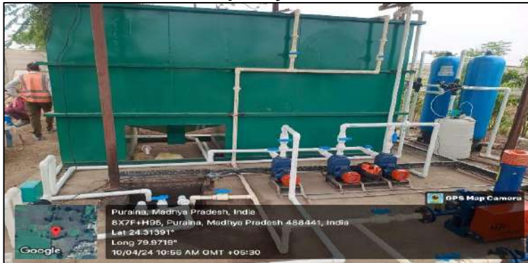
STP With Capacity 25 KLD
