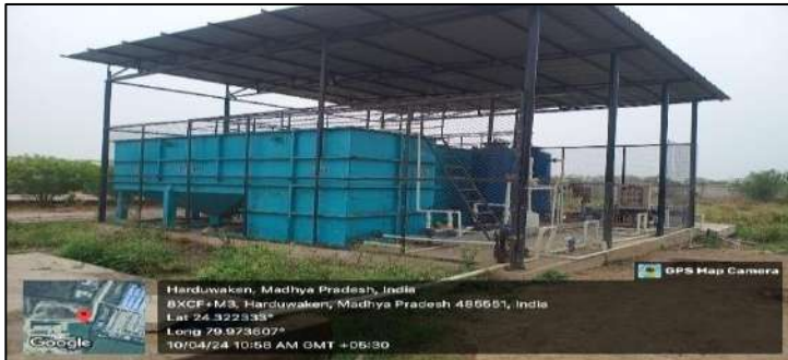
STP With Capacity 25 KLD
