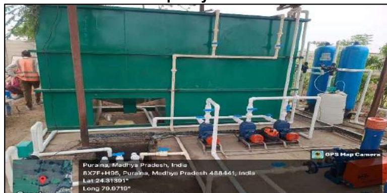
STP With Capacity 25 KLD
