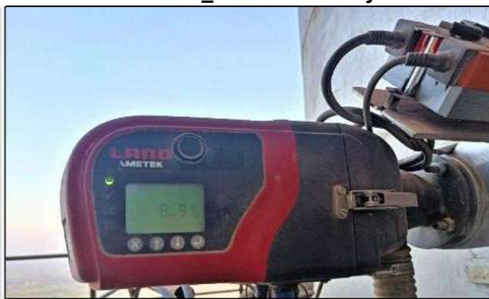
Raw _ Mill Stack Analyser
