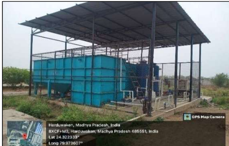
STP With Capacity 300KLD
