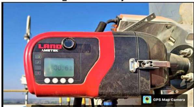
Cooler _ Mill Stack Analyser
