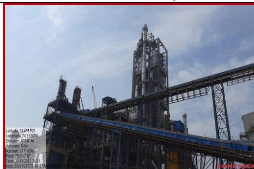
Raw material covered belt conveyor
