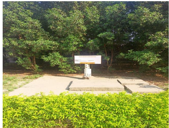
Rain Water Harvesting Pit No-1
