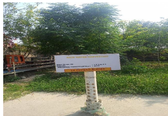
Rain Water Harvesting Pit No-3
