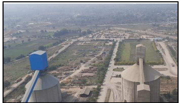
Clinker Storage Silo
