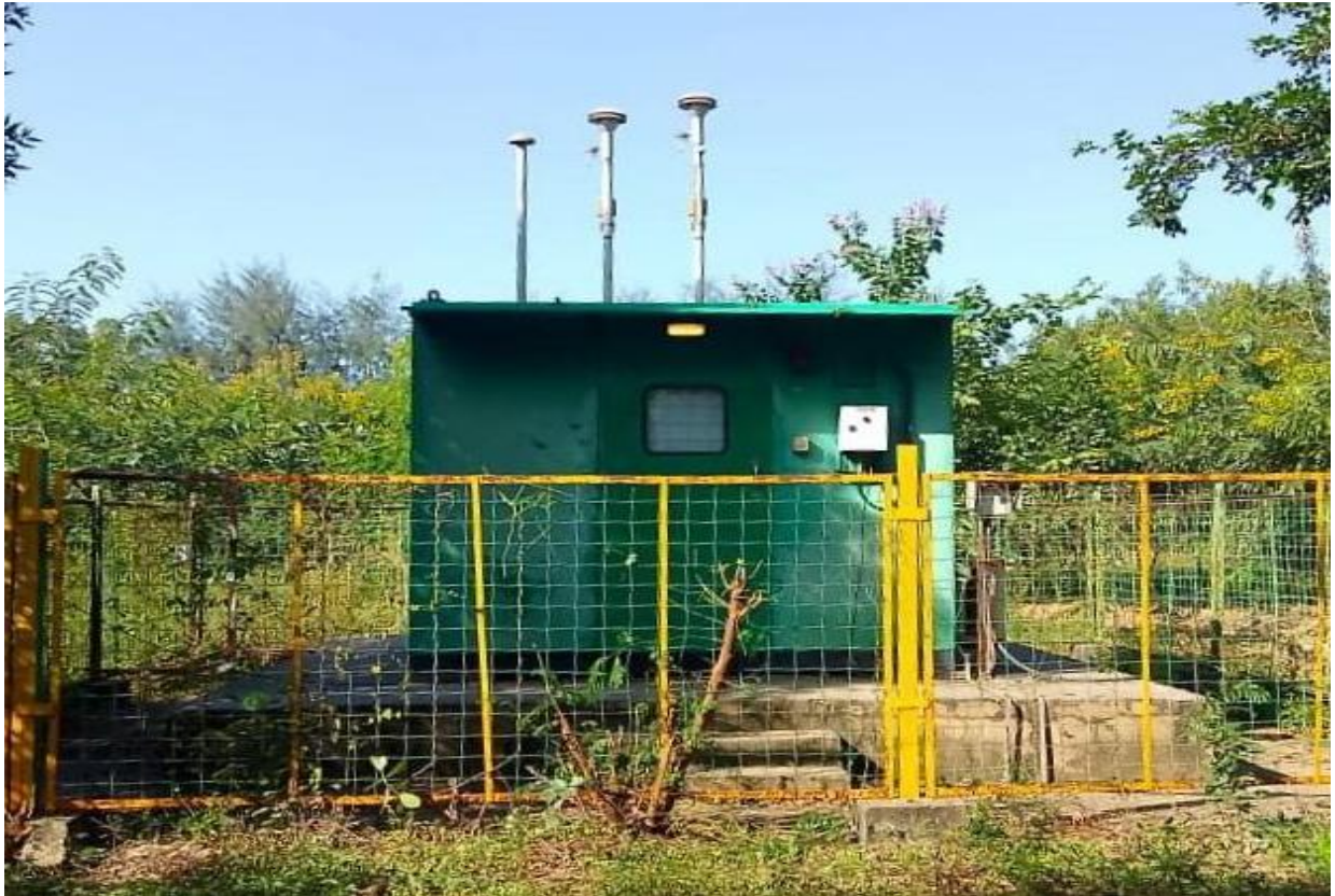
Continuous Ambient Air Quality Monitoring Station (CAAQMS)
