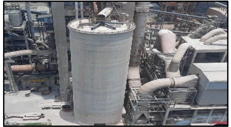
Raw mill storage in CF silo
