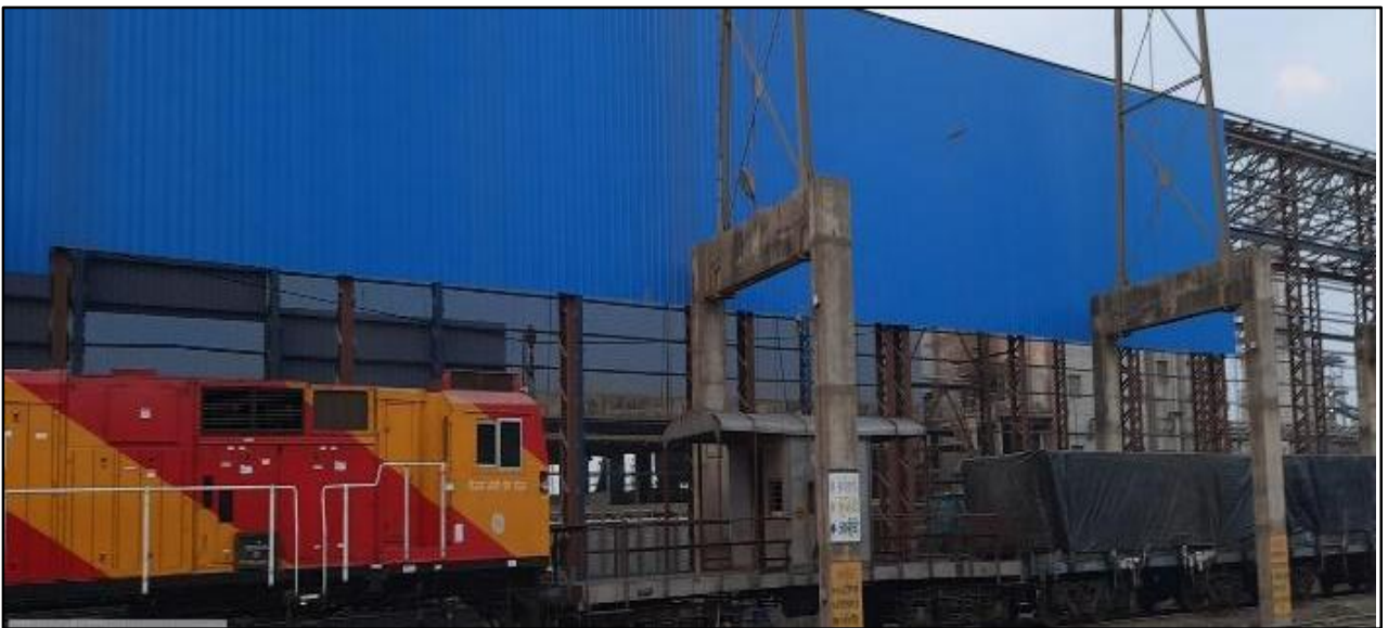
Material Transportation by railway
