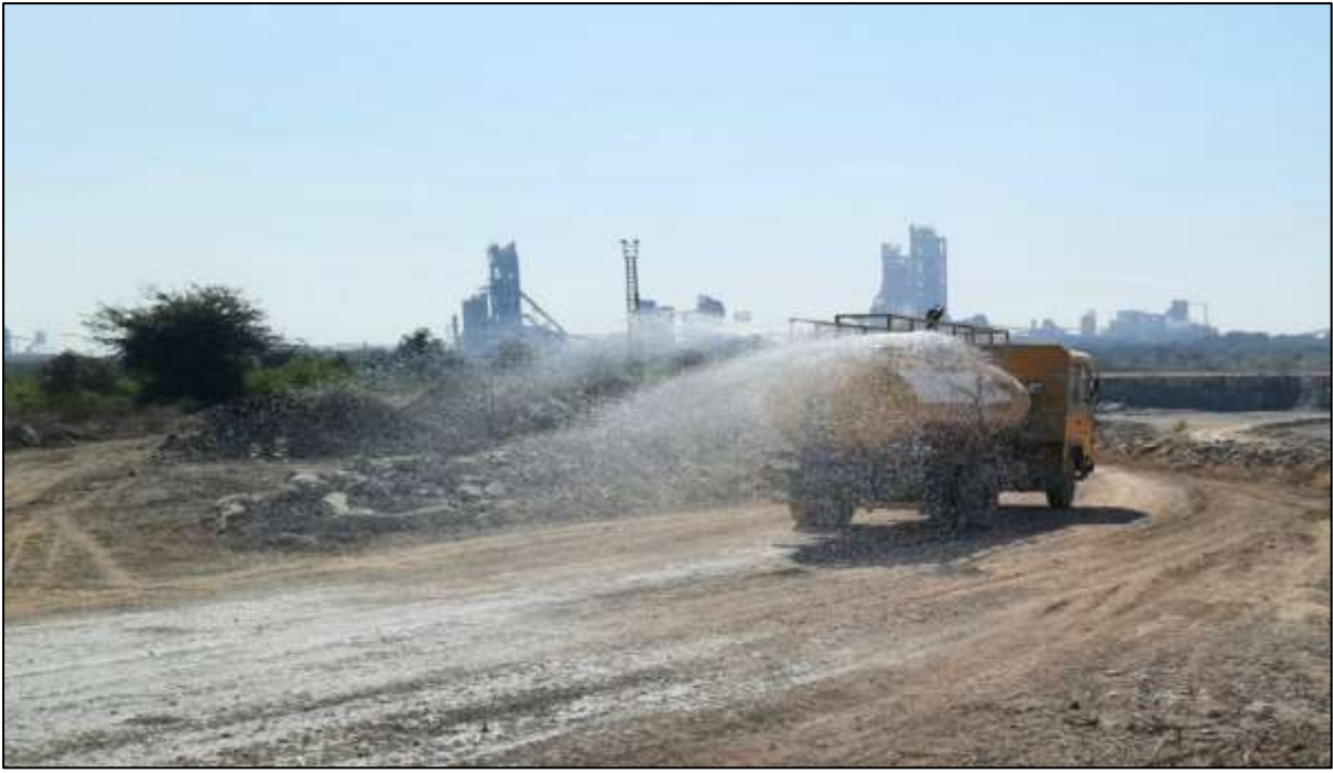
Sprinkling Water on Haul road
