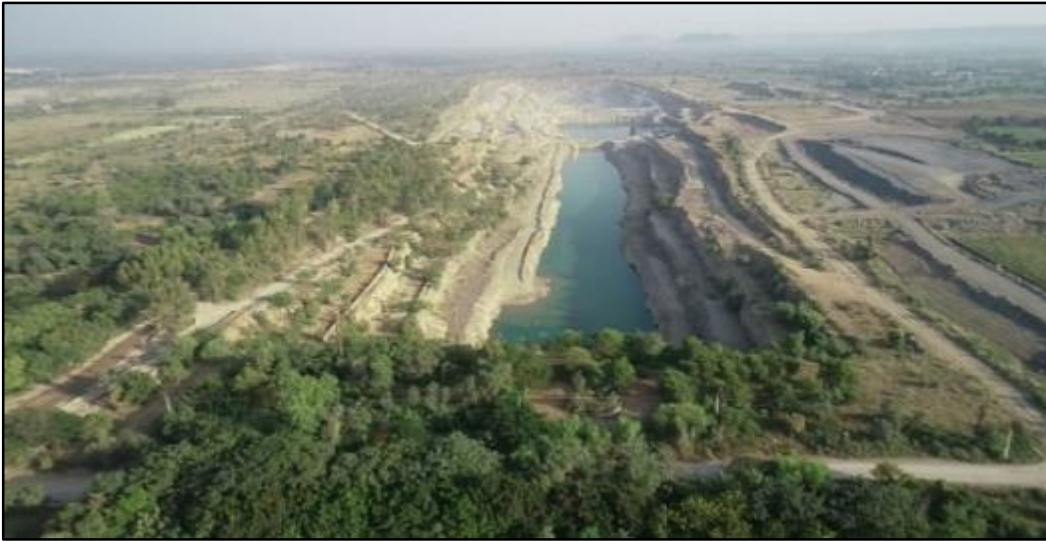
Rain Water Harvesting through Mine Pit-2 (South Pit)
