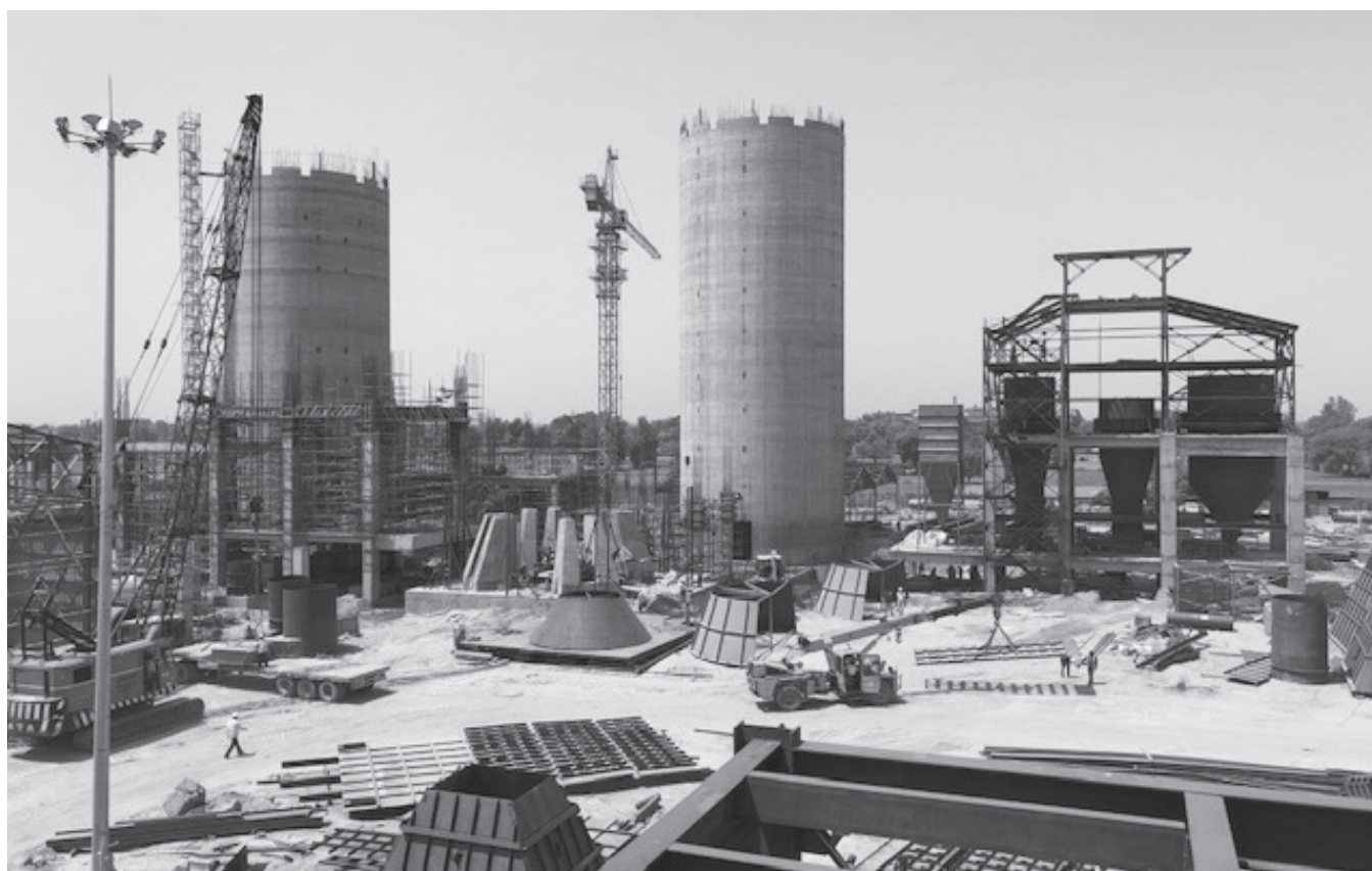
Aligarh Grinding Unit (Greenfield Expansion)
