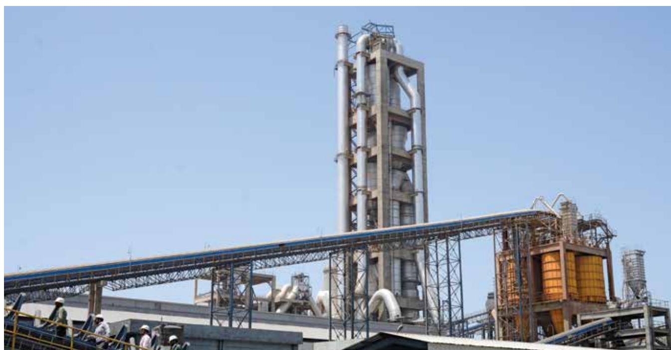
A view of Mangrol plant
