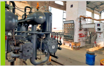
Commisioning of oxygen genration & filling plant An oxygen plant of 80 m 3 /hour capacity was installed and commissioned at the Panna plant of JKCement.
