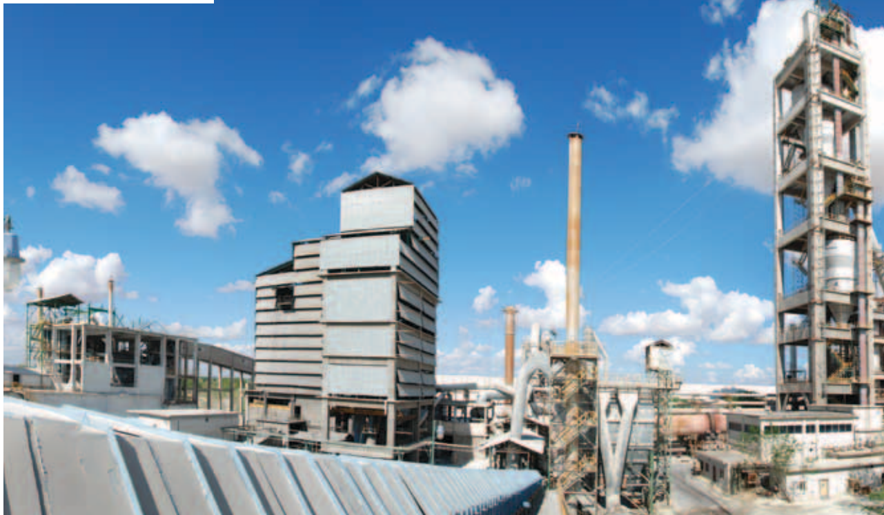
White Cement Plant at Gotan
